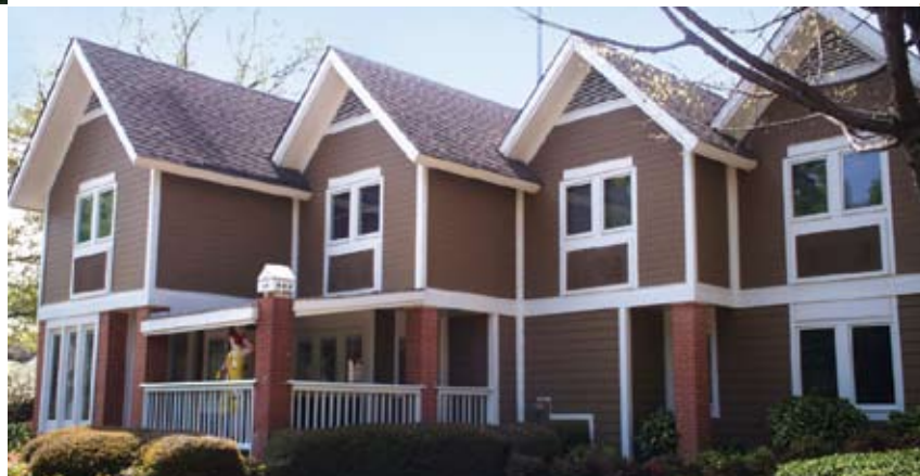
Left: The Dan Rawls Company completely renovated and currently maintains the Ronald MacDonal House in Greenville, S.C.
